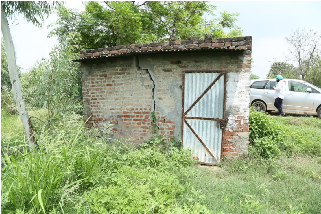
Structures in Land proposed for Acquisition
